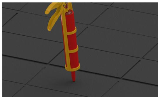
Filling the pilot hole with sealant is a secondary waterproofing step, which is required by the roofing manufacturers.
