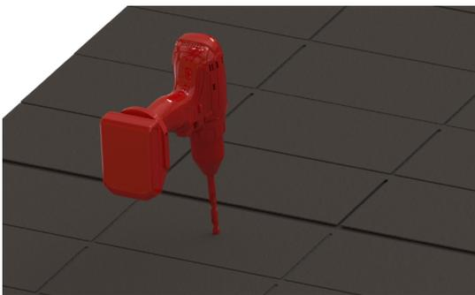
Drill a 1/4" pilot hole by drilling square to the rafter using a 1/4" drill bit.
